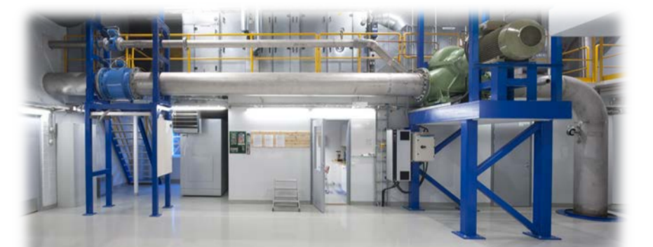
Figure 4. Entrance hall of the flow laboratory.
